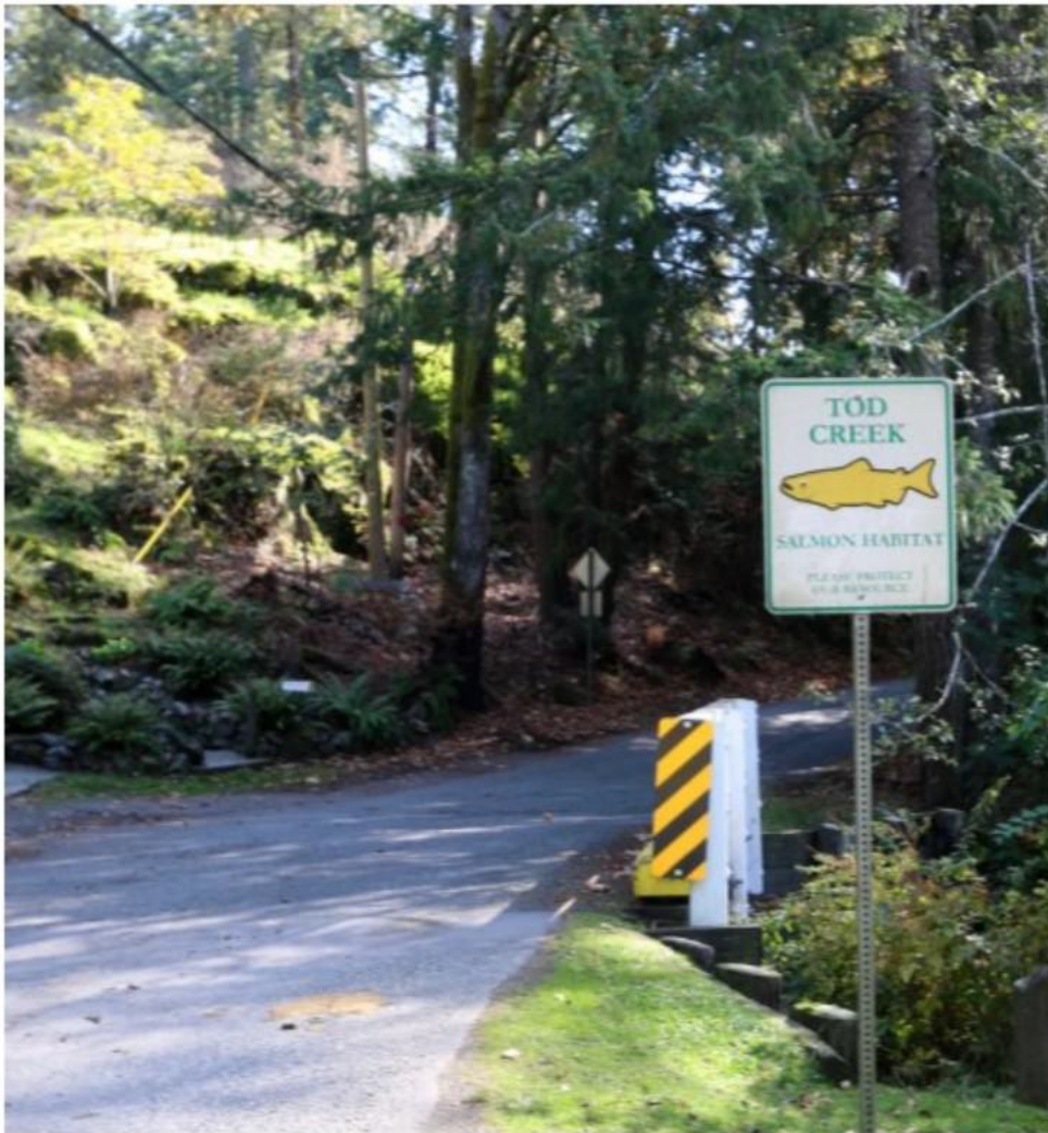
Bridge over Tod Creek, Goward Road
