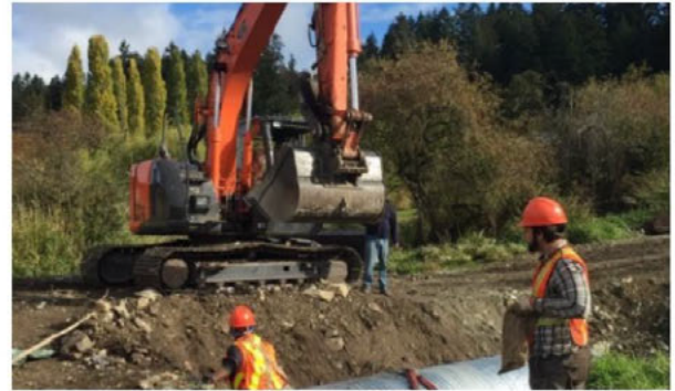
Digging and setting the channels
